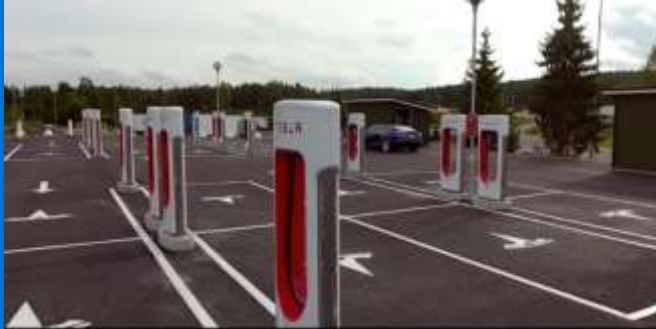
World largest fast charging site (Norway, 20 x 120 kW (2.2 MW total)
